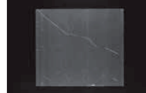
Surface reflection is reduced and a clear image of the damage can be made.
